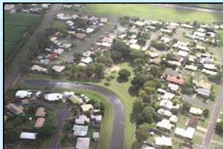
Woongarra Irrigation Channel
