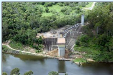
Isis Pump Station
